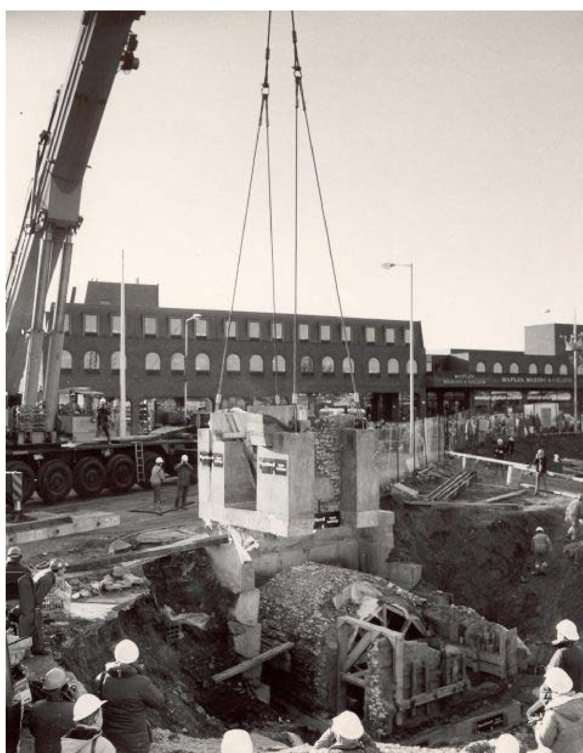
Excavation of the Undercroft, 1986
