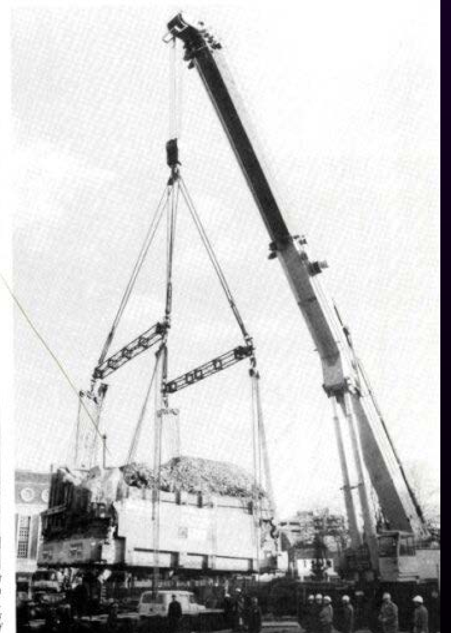
Above, a workman positions chains to lift the main part of the undercroft, which weighs 70 tons. Right, the fragile structure, which has been underpinned to protect it, is ready to be transported through the streets of
